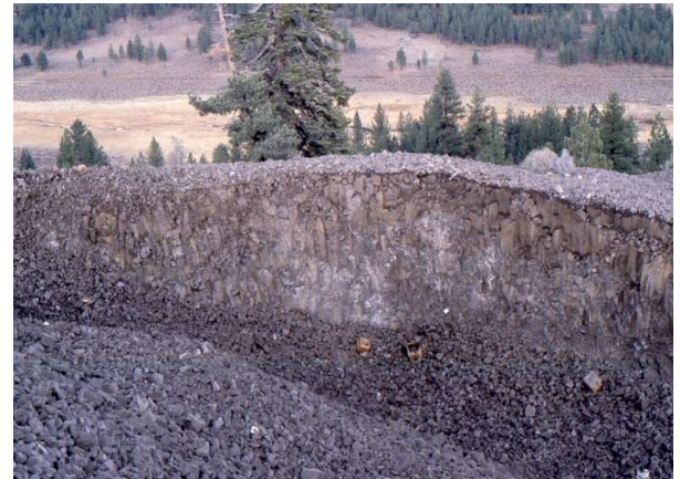
Photo 6 - The east wall where the ridge line has been preserved. Fragmentation is typical for entire shot.
