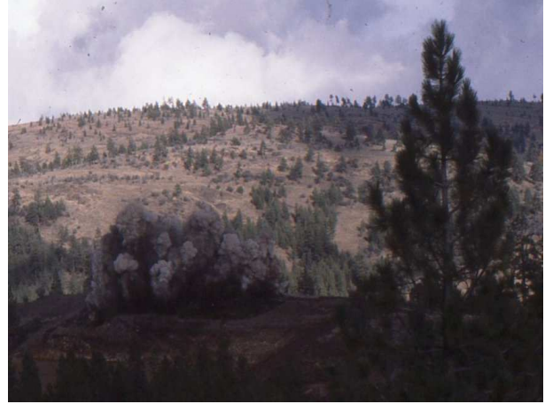
Photo 4 - Opening holes and the next two or three delays have detonated.
