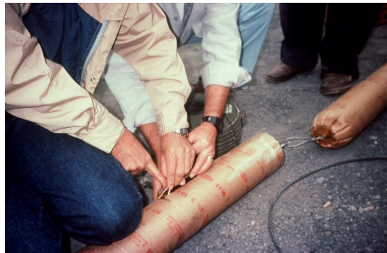
Photo 2 – Ed and Wes inserting caps.
